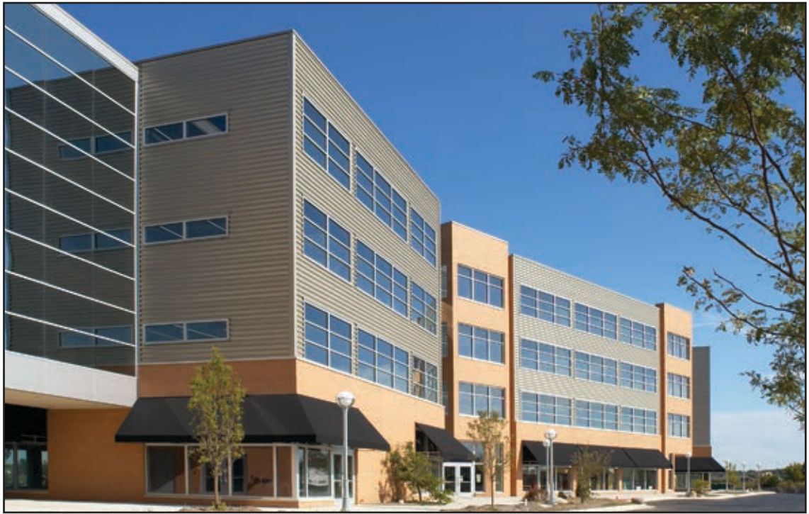
Project: Perryville Place Location: Rockford, IL Architect: David Hagney AIA and Barrett Studio Products: Mega-Rib in Bare Galvalume
