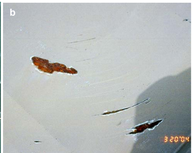
Figure 9. Photographs of paint abrasion damage on the major rib of the panel (a), and scratches on the surface of a painted panel resulted in premature corrosion (b).
