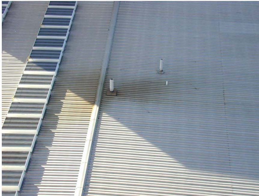
Figure 34. The bare GALVALUME® roof was corroded around the laboratory vent.
