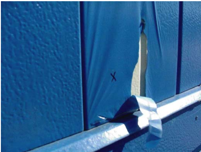
Figure 48. The topcoat delaminated from the primer.
