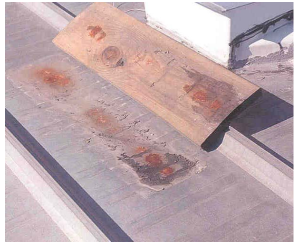
Figure 31. Corrosion occurred under the treated lumber because chemicals, particularly copper compounds, leached from the wood accelerating the corrosion.
