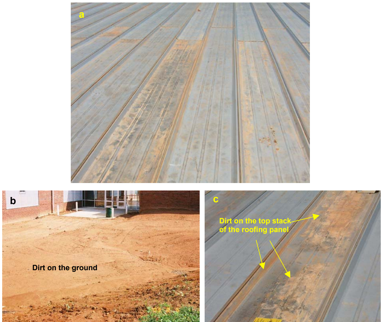
Figure 1. Photographs of stains and inconsistent appearance of a bare GALVALUME® roof (a), dirt on the ground at a building site (b), and dirt concentrated on the roofing panels on the top of the stack (c).
