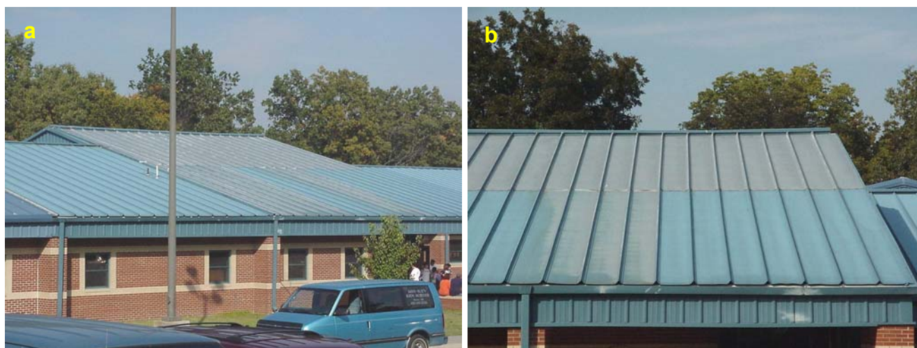
Figure 44. Non-uniform fading of a prepainted roof with noticeable differences in color from one section to another section (a) and its close look (b).
