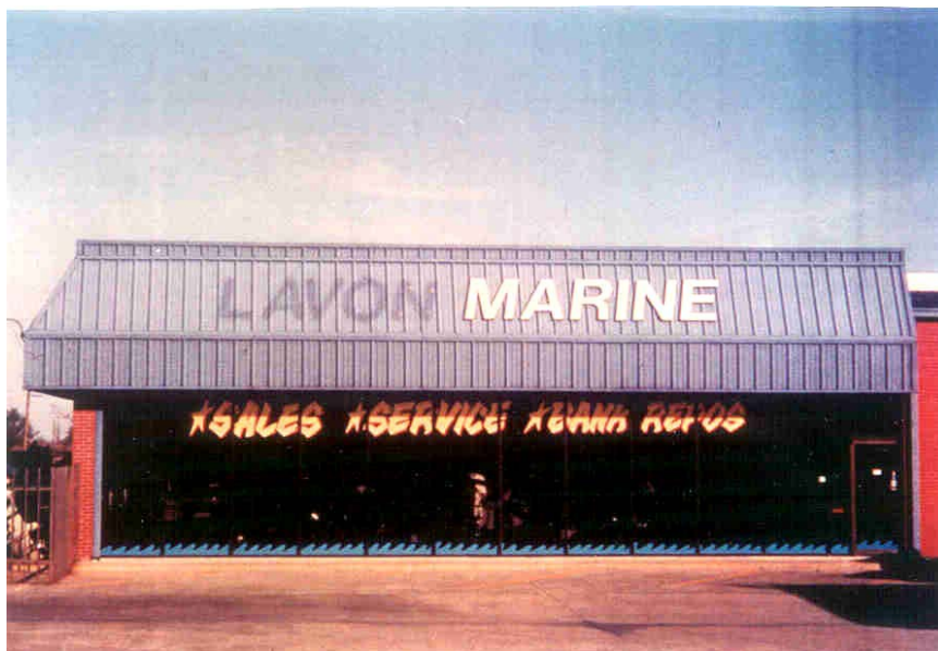
Figure 43. Color fading of the paint on prepainted panels due to UV light from the sun.
