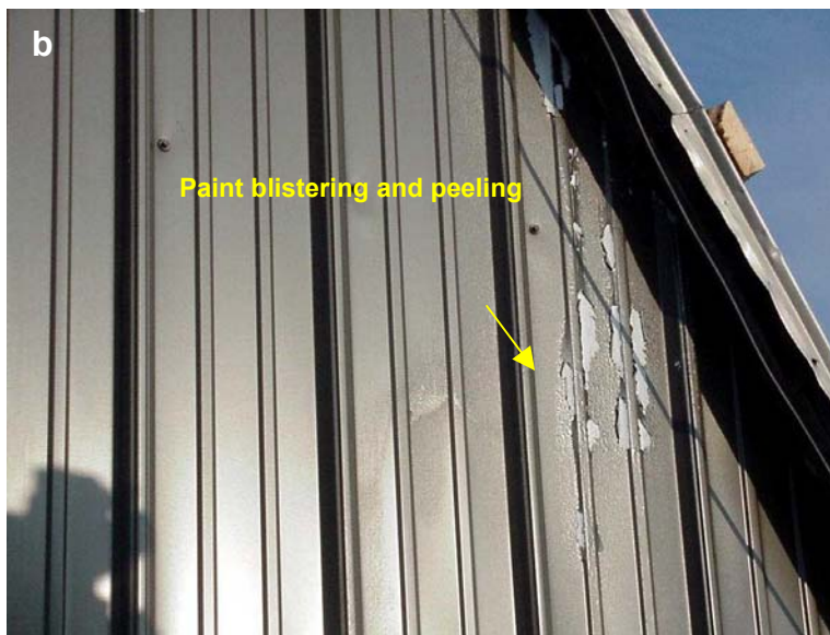
Figure 5. Photographs of wet storage stains on bare galvanized steel siding (a), and wet storage causing paint blistering and peeling on prepainted galvanized steel siding (b).
