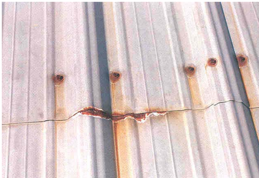
Figure 24. Crevice corrosion caused by poor end lap sealing on a GALVALUME® roof.
