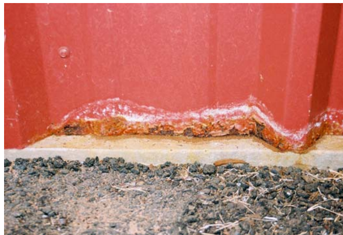
Figure 18. Premature corrosion at the bottom edges of the prepainted GALVALUME® panel caused by direct contact with the concrete foundation.
