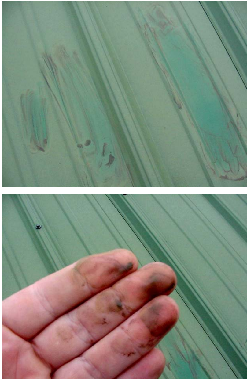
Figure 38. The prepainted GALVALUME ® roof panel discoloration is due to dirt coverage.
