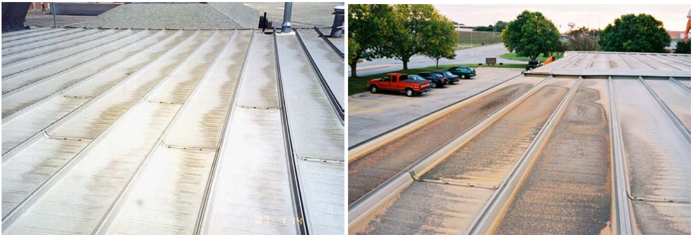
Figure 22. Photographs of water ponding on a GALVALUME® roofs due to improper slope of the roof.
