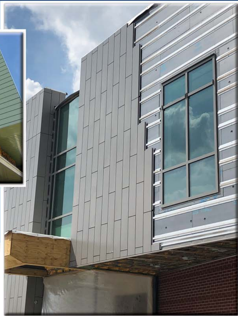
F-Series installation over hat section sub-framing.
