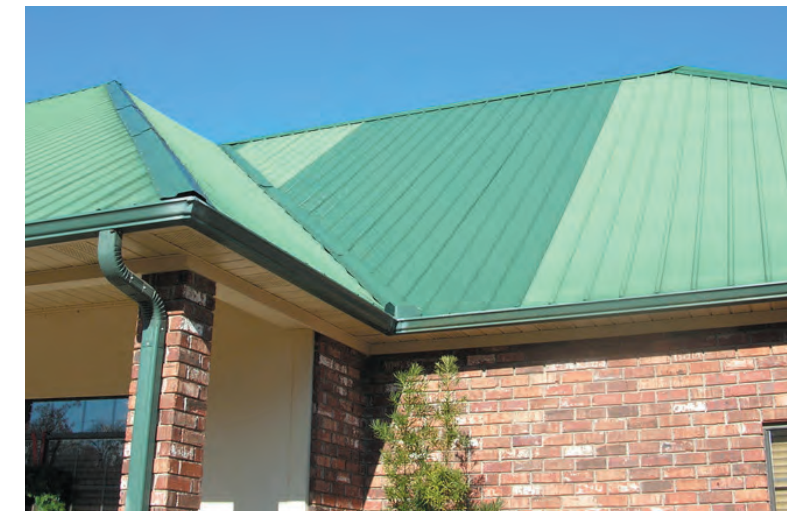
Both Kynar 500 (PVDF) and Silicone Modified Polyester (SMP) panels were installed on this Louisiana residence pictured above. On day one, colors were identical. Less than 8 years later, the Silicone Modified Polyester (SMP) panel shows fading and chalking. Note, no fade or chalking of the darker Kynar 500 (PVDF) panels.
