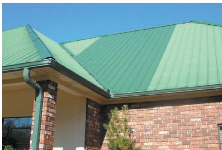
Both Kynar 500 (PVDF) and Silicone Modified Polyester (SMP) panels were installed on this Louisiana residence pictured above. On day one, colors were identical. Less than 8 years later, the Silicone Modified Polyester (SMP) panel shows fading and chalking. Note, no fade or chalking of the darker Kynar 500 (PVDF) panels.
