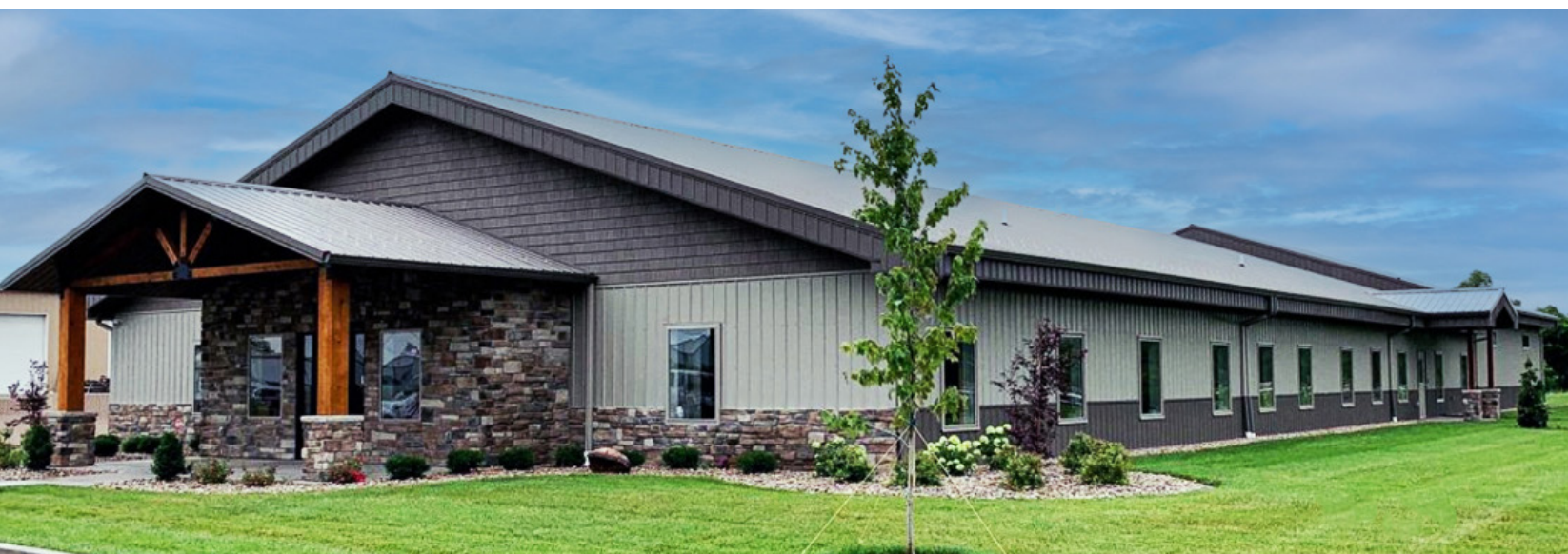
Photo Courtesy of Blunier Buildings
