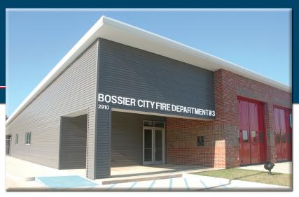
Available in both fixed and floating systems, McElroy Metal's Wave panels are concealed fastener wall panels that can be installed vertically or horizontally over solid substrate or subframing. Wave Fixed is installed with Wave's integral fastening flange which is roll formed into the panel during the manufacturing process and can be utilized for panels length 40' or less. Wave Floating panels utilize separate clips and should be specified for panel lengths 40' or greater.
