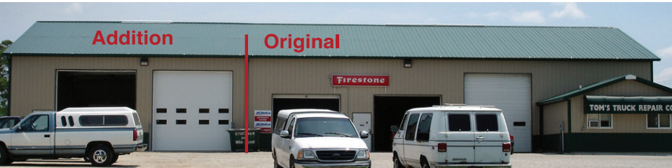
Building addition dramatically illustrates Kynar 500 (PVDF) superior performance. This building was built in two phases, nine years apart. Note, no color difference in the two halves of the roof. No fade! No chalk!
