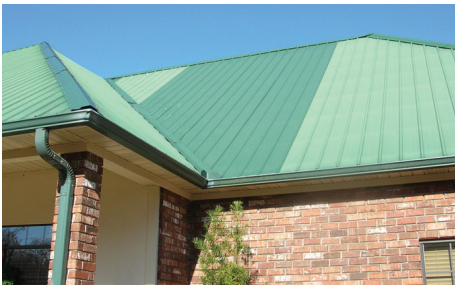
Both Kynar 500 (PVDF) and Silicone Modified Polyester (SMP) panels were installed on this Louisiana residence. On day one, colors were identical. Photo taken less than eight (8) years later shows fading and chalking of the lighter Silicone Modified Polyester (SMP) panels. Note, no fade or chalking of the darker Kynar 500 panels.
