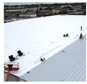
R-Seal is designed to be installed on top of open frame ۲ metal buildings with purlins spaced 5' O.C.
