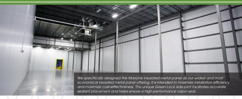
Panel Use Partition Wall, Liner Wall, Tee Supported Ceiling
